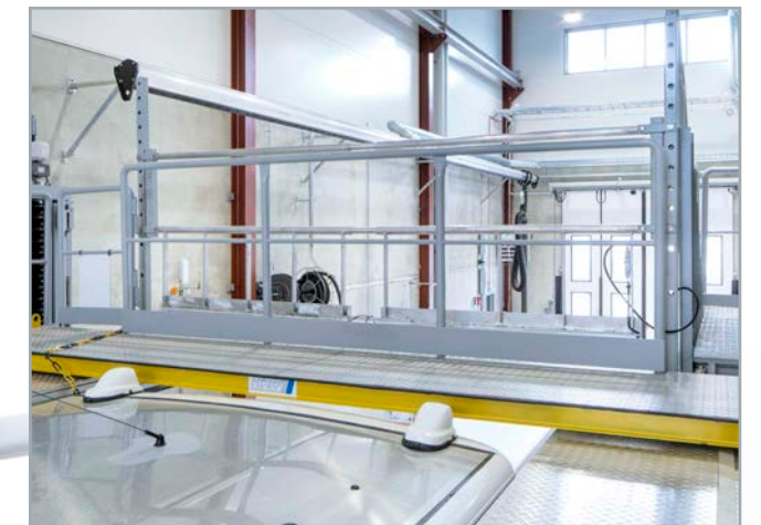
Safety equipment at the ends of the platforms: Adaptable to the length of the buses.
