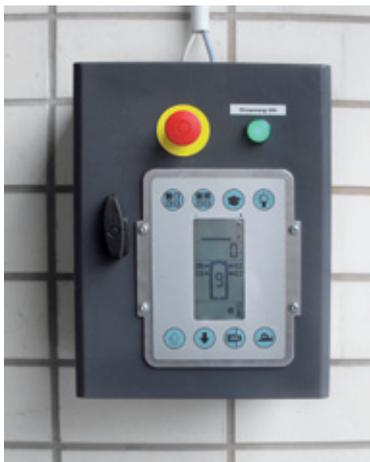
We recommend to install the power unit outside of the washing area.
