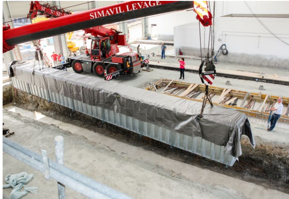
When installing a cassette the concrete base needs to be 150mm thick and 1500mm wide
